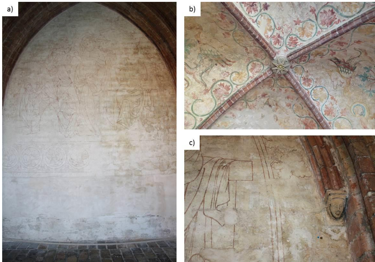
Figure 1: Photographs from the Schwahl in Schleswig. a) bay no. 5 showing the murder of innocents in Bethlehem b) example for the polychrome decorated vaults c) detail of bay 5 with an extreme presence of yellowish encrustations on its surface.
